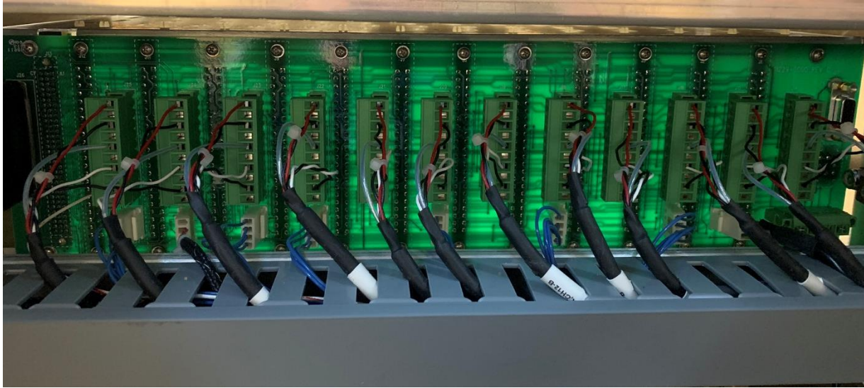
Figure 13: Detectors terminated directly to IA, bypassing FITA
